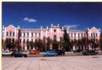
Education and Research Institute of Mechatronics and Management Systems building
